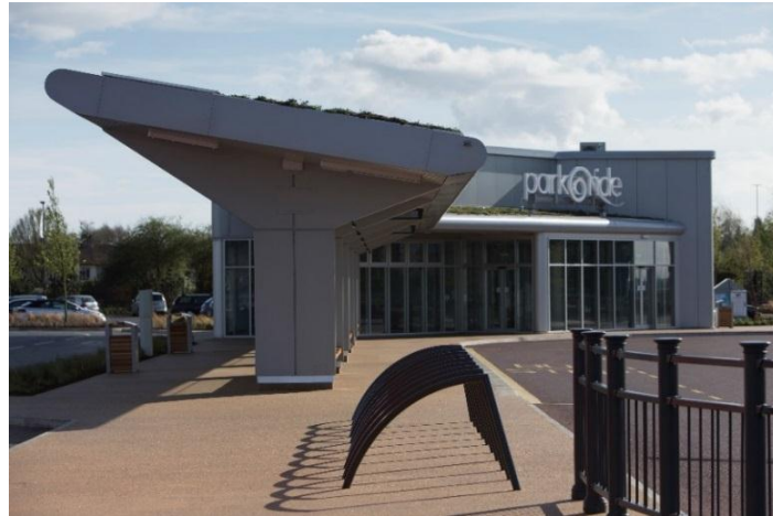
Park & Ride terminal building at Tipner
